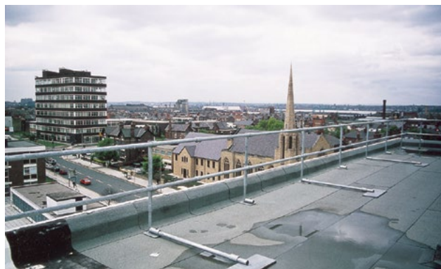
Figure 40 Permanent guard rail retrofitted during refurbishment work. Similar protection can be included in initial designs (image courtesy of Safesite Limited)
