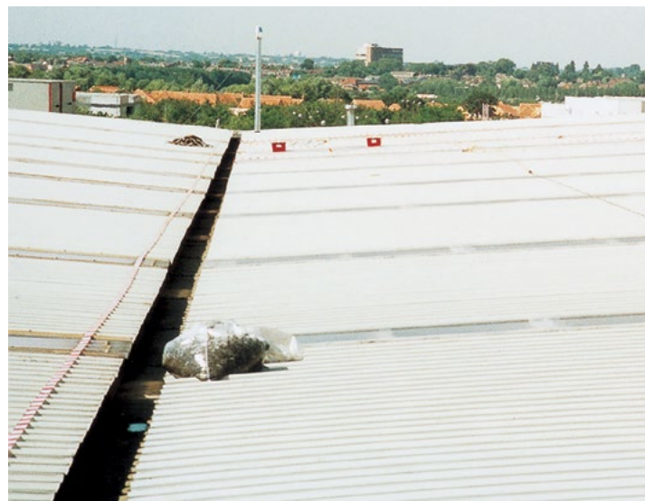
Figure 27 In some light conditions, it is difficult to distinguish the roof lights from the metal sheets on this type of roof. The valley gutter is very narrow and the roof lights extend down to gutter level. Both of these features increase the risk during cleaning, maintenance and refurbishment
