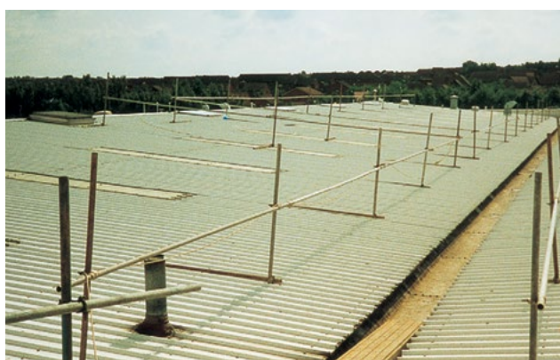
Figure 20 Demarcation barriers on a large, non-fragile roof preventing access to the adjacent roof lights. The roof lights are at least 2 m from the barrier
