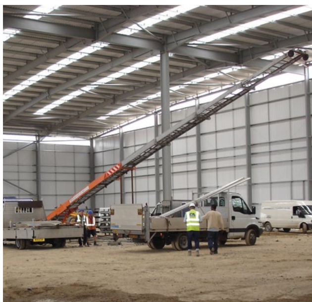
Figure 35(a)–(c) Mechanical handling of large roof sheets (images courtesy of Advisory Committee on Roof Safety)
