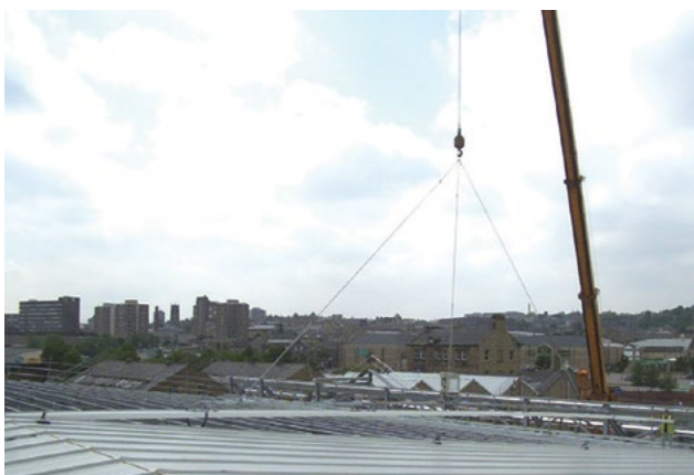
Figure 36 (a)–(c) 24-m long roof panels being mechanically lifted from ground level and installed on roof
