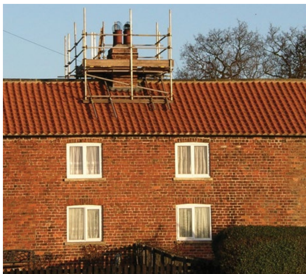
Figure 24 A traditional chimney scaffold
